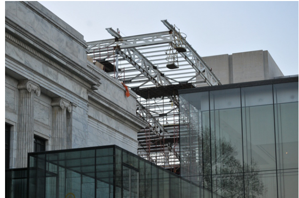
Top to Bottom: 1. CMA skylight steel erection 2. CMA skylight steel erection
