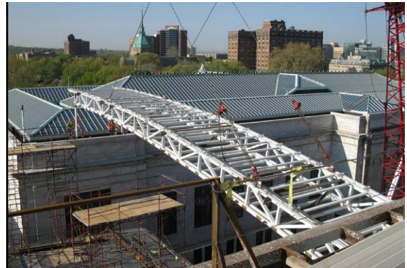
Top to Bottom: 1. CMA skylight steel erection 2. CMA skylight steel erection
